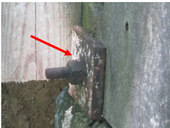
Photo 5. Tie-rod Washer is Positive for Lead.
