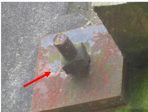
Photo 5. Orange Tie-rod Washer is Positive for LBP.
