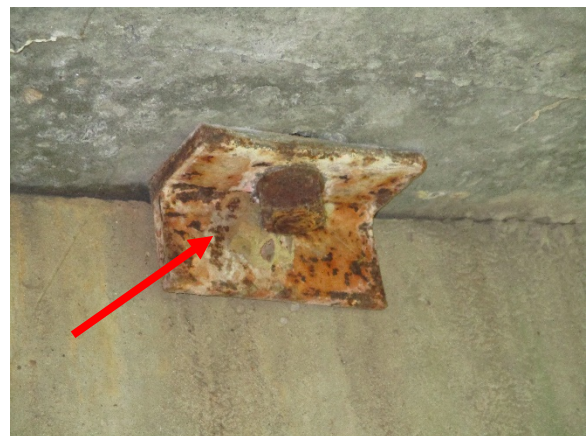
Photo 6. Orange L-Bracket is Positive for LBP.
