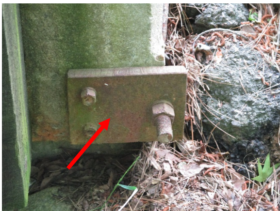
Photo 5. Tie-rod Washer is Positive for Lead.
