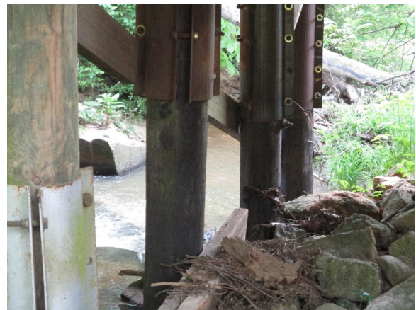
Photo 4. Metal Sleeve on Timber Pile.
