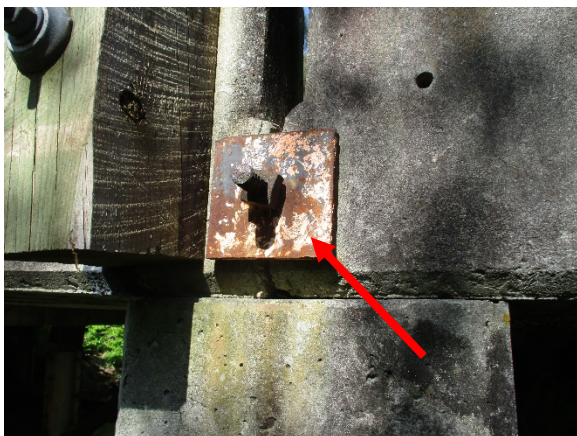
Photo 5. Tie-rod Washer is Positive for Lead.
