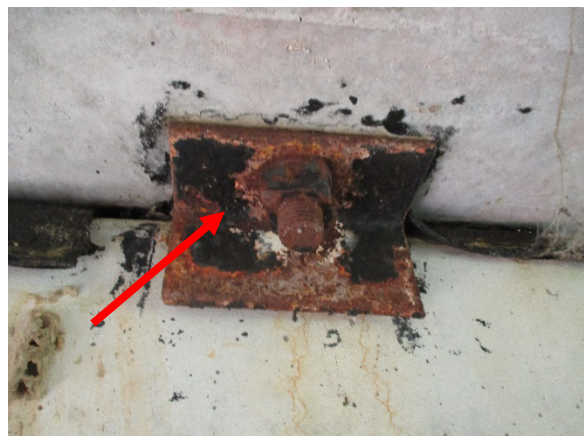
Photo 6. L-Bracket is Positive for Lead.
