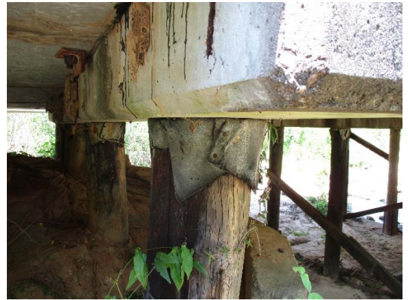
Photo 4. Timber Pile Cap Felt
