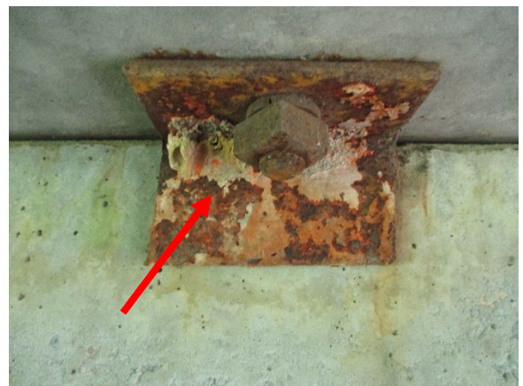
Photo 6. L-Bracket is Positive for Lead.
