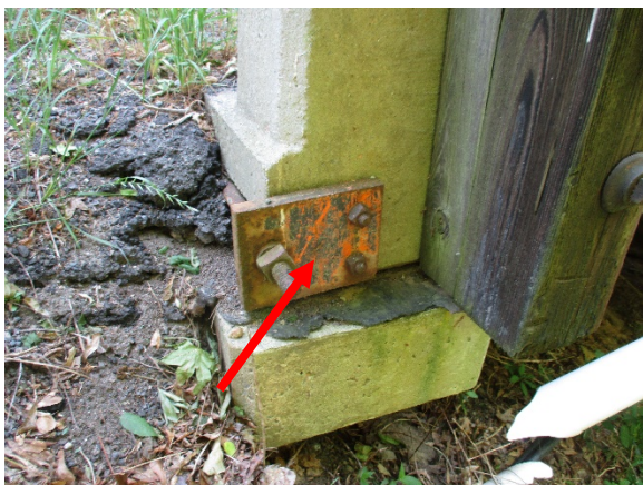
Photo 5. Orange Tie-Rod Washer is Positive for Lead.
