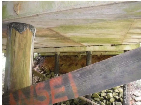
Photo 4. Timber Pile cap Felt.
