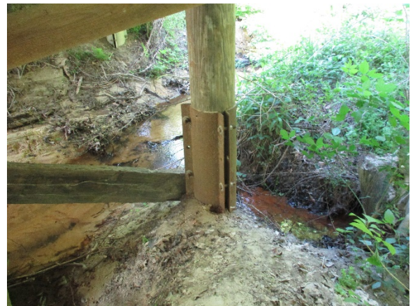
Photo 4. Metal Sleeve on Timber Pile.
