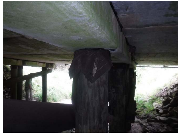
Photo 4. Timber Pile Cap Felt
