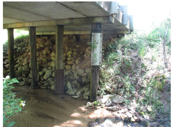
Photo 4. Metal Sleeve on Timber Pile.
