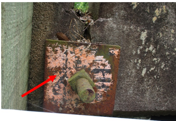
Photo 5. Tie-rod Washer is Positive for Lead.
