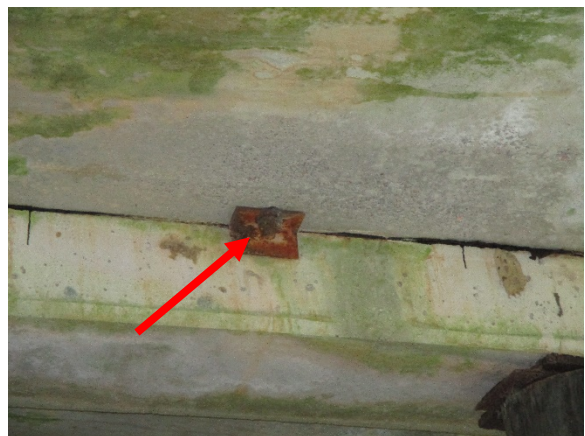
Photo 6. Orange L-Bracket is Positive for Lead.
