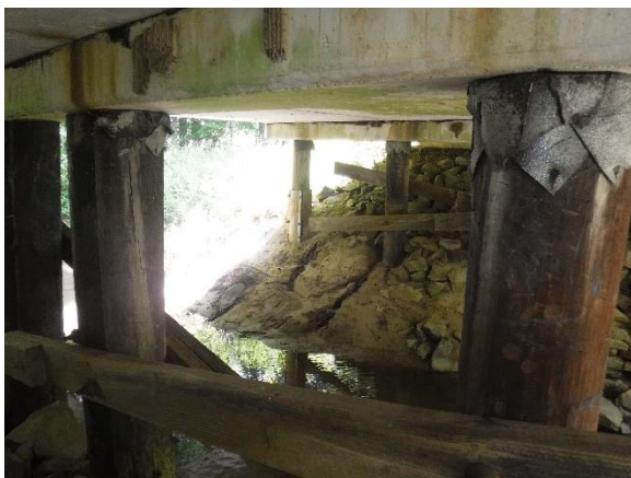
Photo 5. Timber Pile Cap Felt
