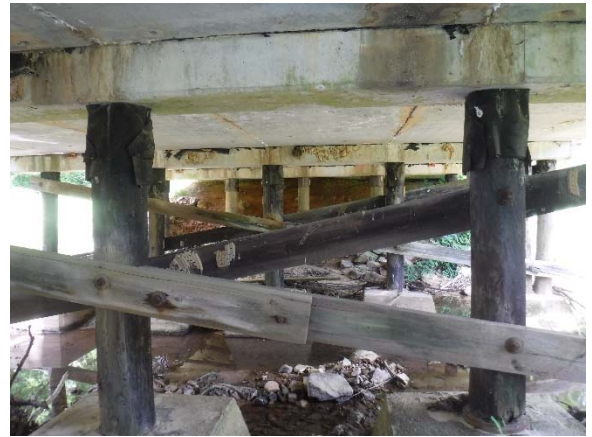
Photo 4. Timber Pile Cap Felt.
