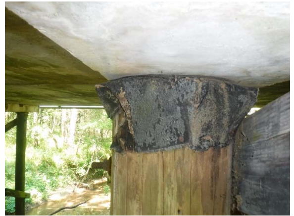
Photo 4. Timber Pile Cap Felt
