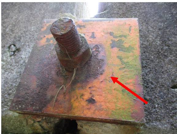
Photo 5. Tie-rod Washer is Positive for Lead.
