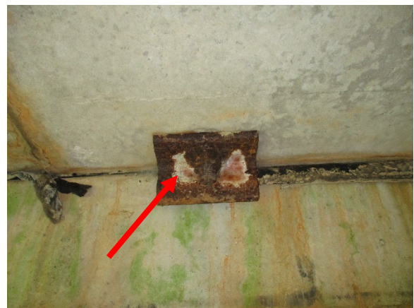
Photo 6. L-Bracket is Positive for Lead.
