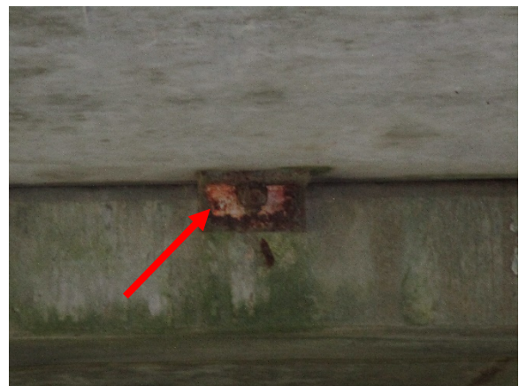
Photo 6. L-Bracket is Positive for Lead.
