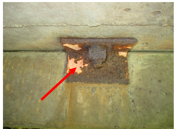
Photo 6. L-Bracket is Positive for Lead.
